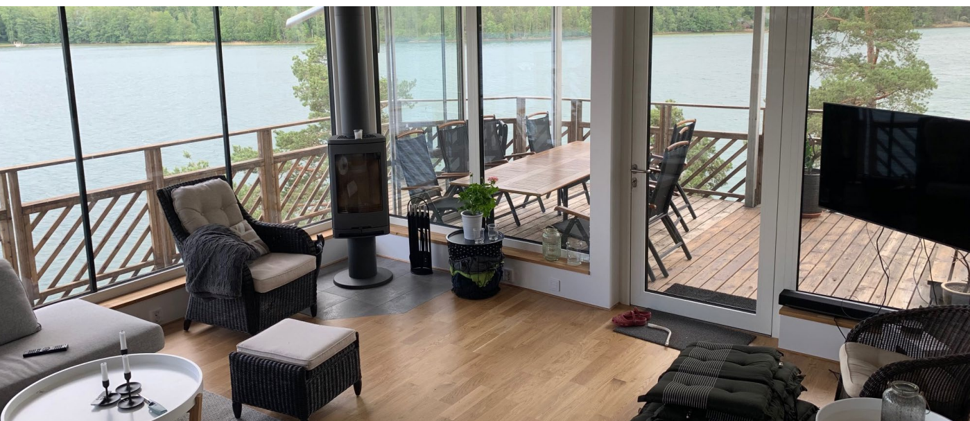
Villa Ola combines laminated ECLAZ x 2 laminated DIAMANT and middle pane VISION-LITE 44.2/16ar/4/16ar/44.8
